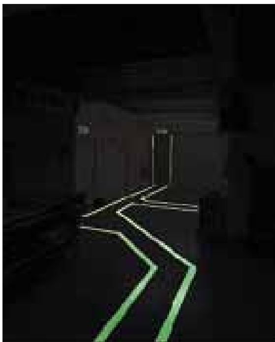
Figure 49: A 'way-guidance' system
