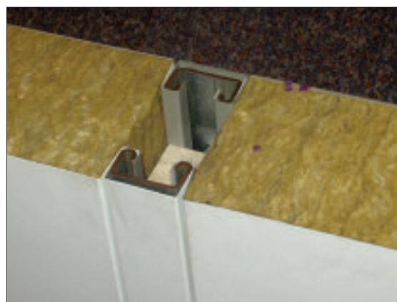
Figure 17: Insulated core panels – internal
