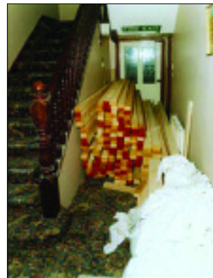
Figure 9: A blocked corridor with incorrect signage
