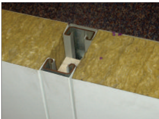
Figure 17: Insulated core panels – internal
