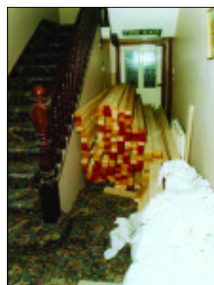
Figure 9: A blocked corridor with incorrect signage
